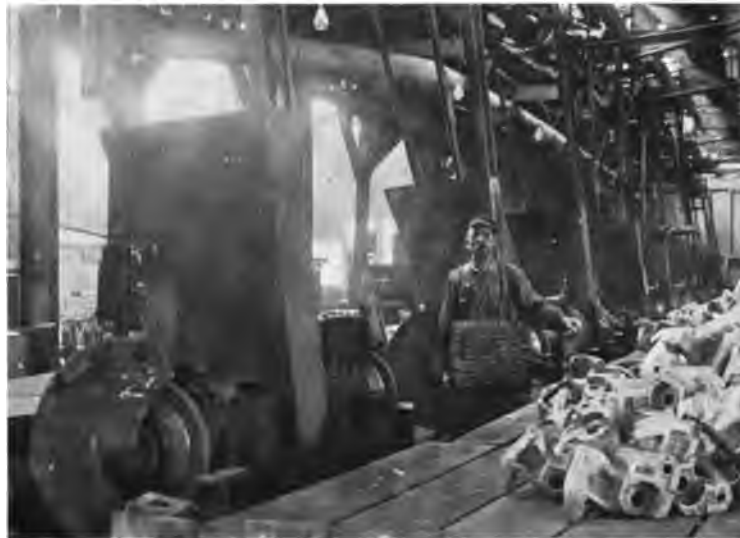
Fig. 4. Department for Snagging Castings. (American Steel Foundries Company.)
